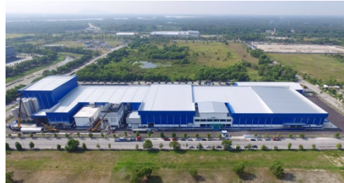
New BOPP plant in Pulau Indah
