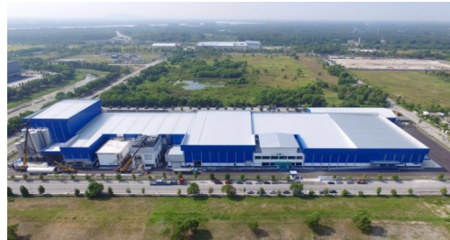
New BOPP plant in Pulau Indah
