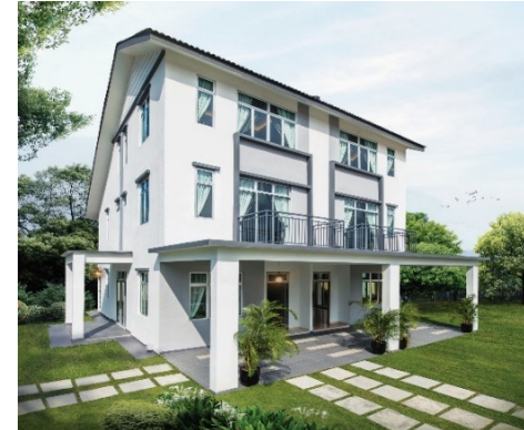
Acacia – 2½-storey terrace houses
