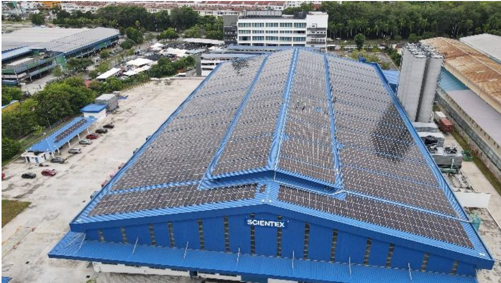
Progress of rooftop solar PV installation at Shah Alam plant
