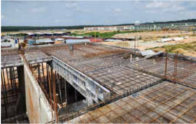
A sample development utilising aluminium formworks
