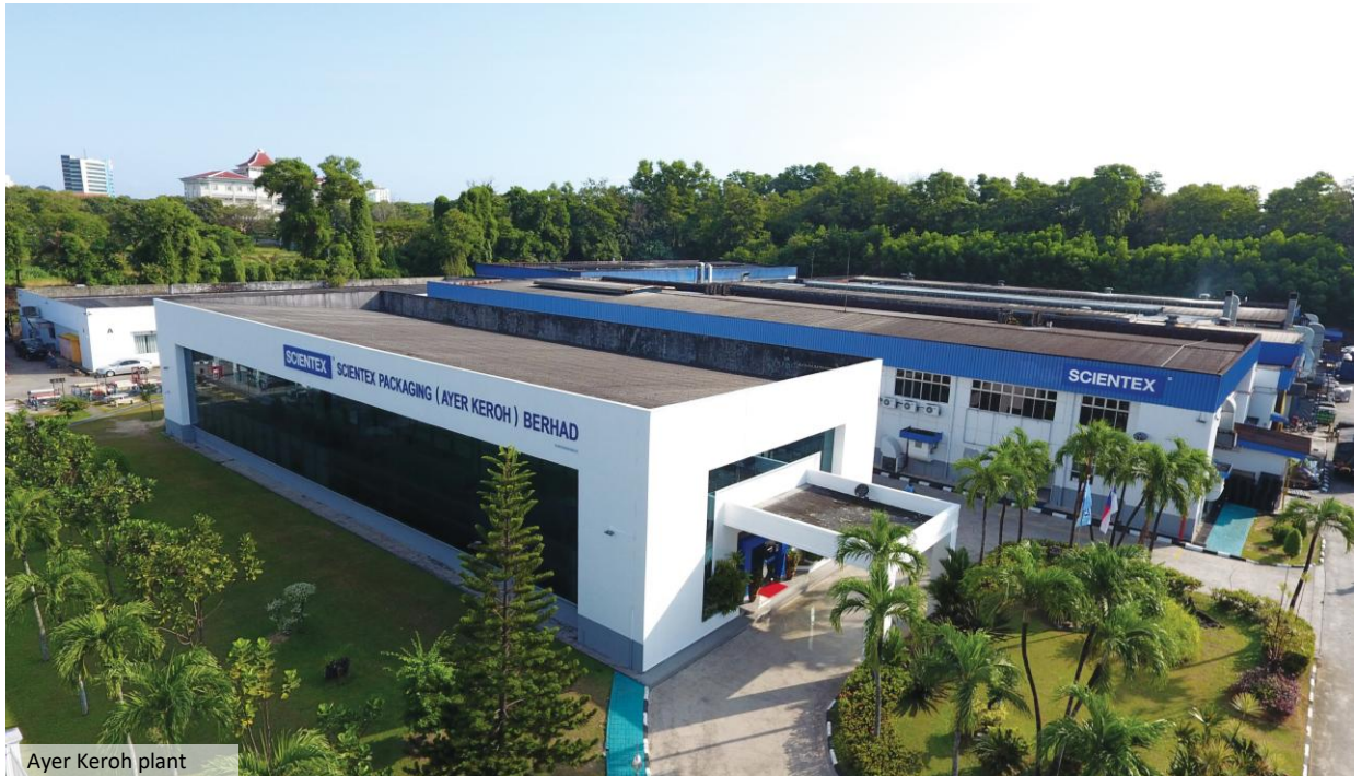
Ayer Keroh plant
