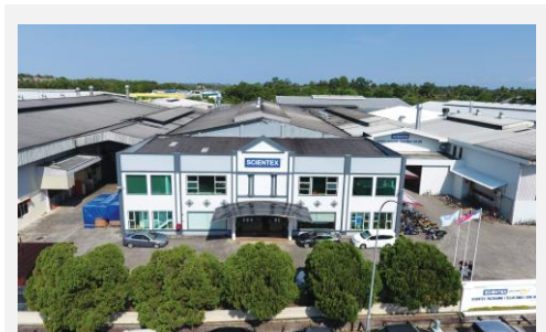
Teluk Emas plant
