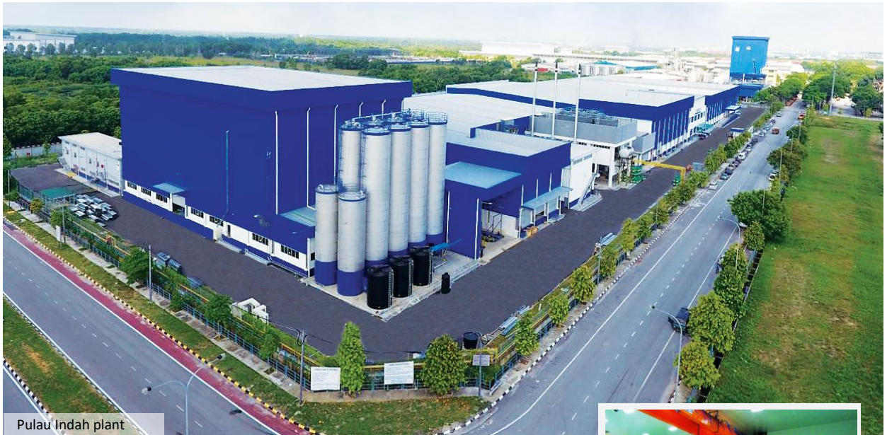
Pulau Indah plant
