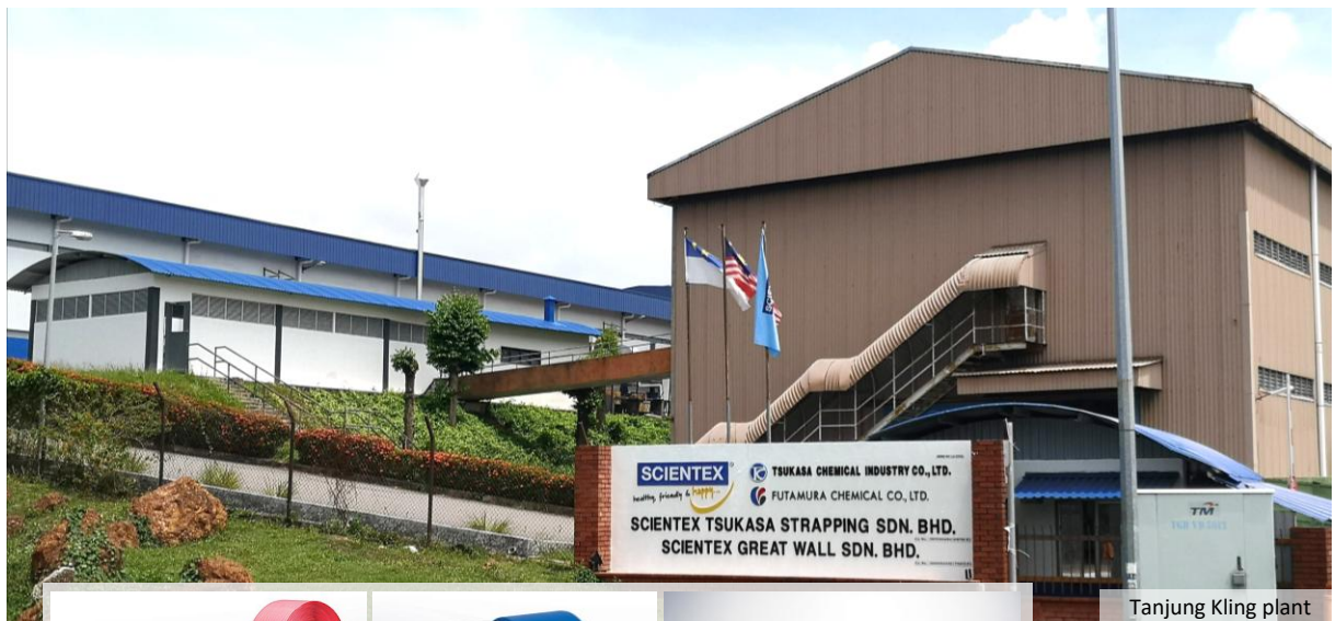
Tanjung Kling plant
