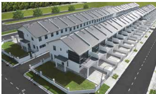
The view of completed double-storey terrace houses at Taman Pulai Mutiara 2
