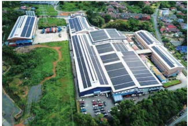
The rooftop solar PV system installed at our plant in Tanjung Kling
