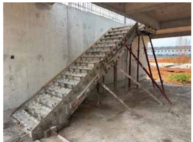
A sample of our staircase aluminium formwork
