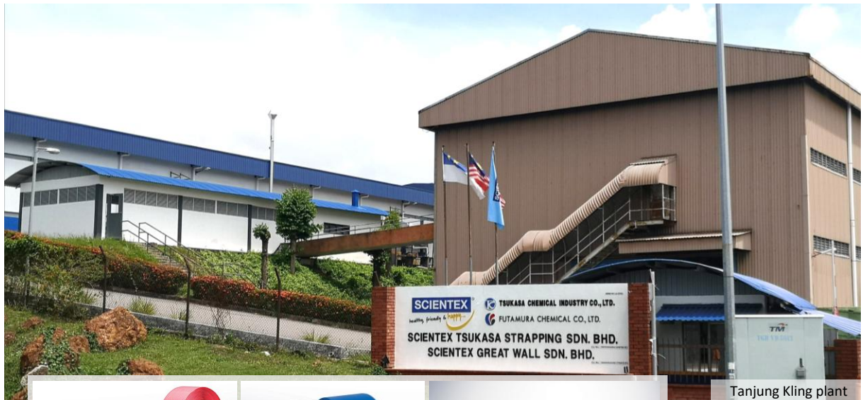
Tanjung Kling plant
