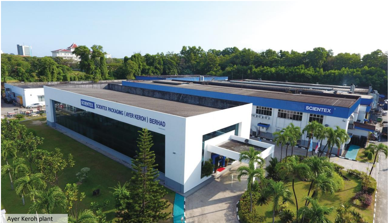
Ayer Keroh plant
