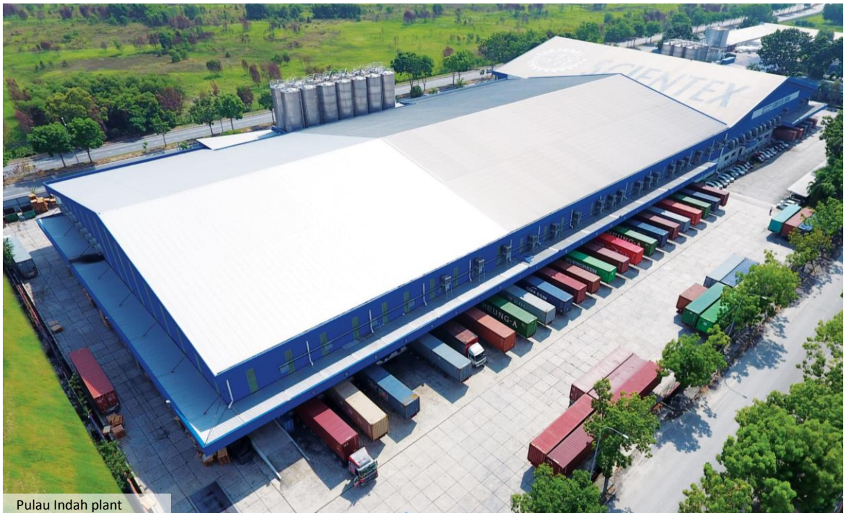
Pulau Indah plant
