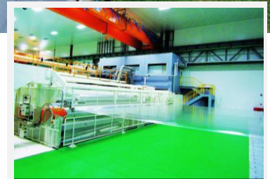
BOPP film stretching plant
