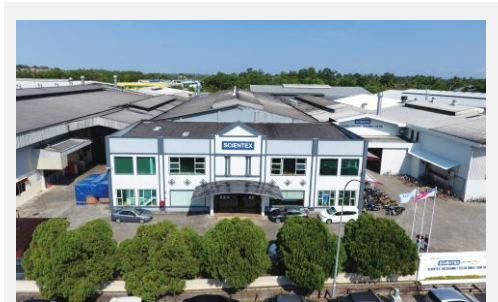
Teluk Emas plant
